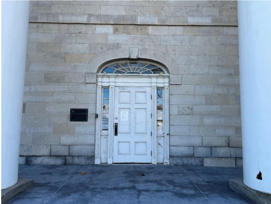
Figure 33: Detail of the primary entrance with original surround and replacement door (A.S.I., 2023).
