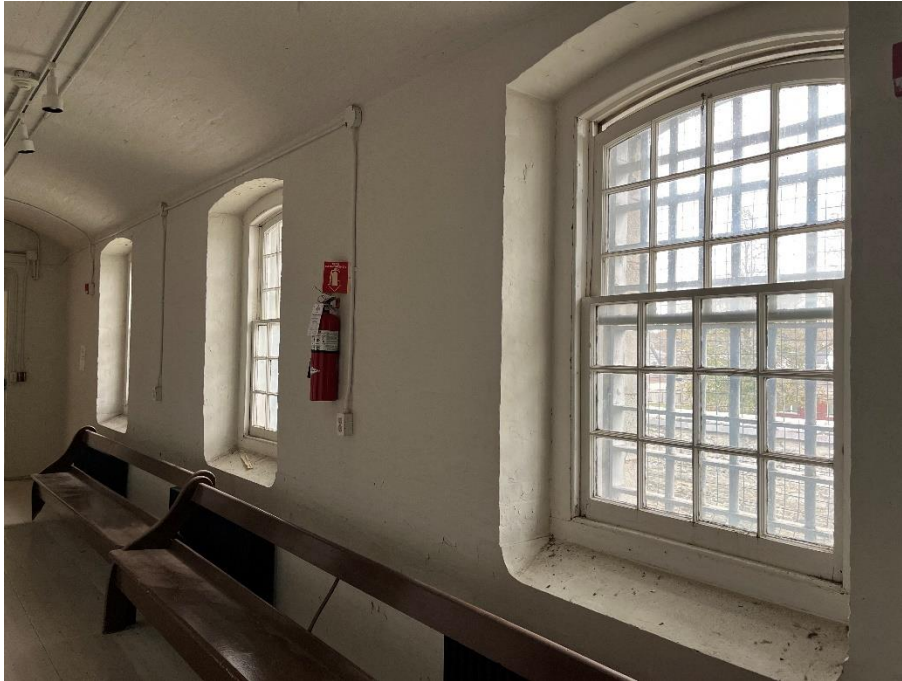
Figure 58: Detail of the 12-over-12 sash windows that are still extant throughout the two-storey building (A.S.I., 2023).
