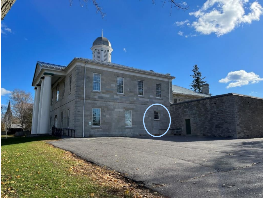
Figure 35: West elevation showing regular placement of window openings, with the exception of one that has been partially infilled (circled) (A.S.I. 2023).
