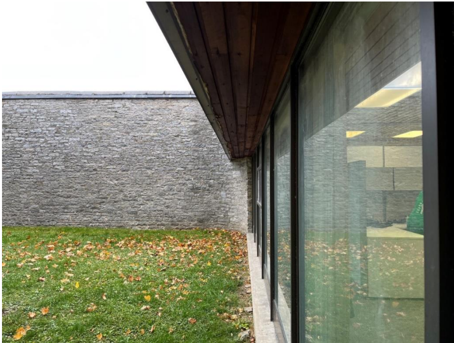
Figure 65: Detail of wood panelled soffit and exterior glazing (A.S.I., 2023).
