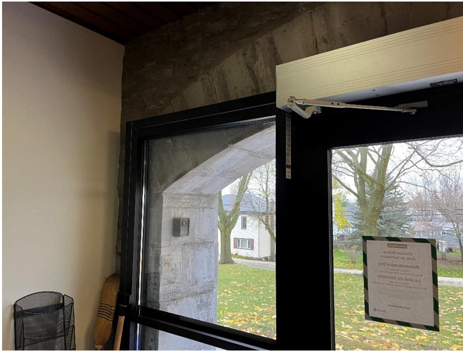
Figure 68: Detail of the placement of the entrance to the Land Registry Office addition against the nineteenth-century opening without altering the opening (A.S.I., 2023).
