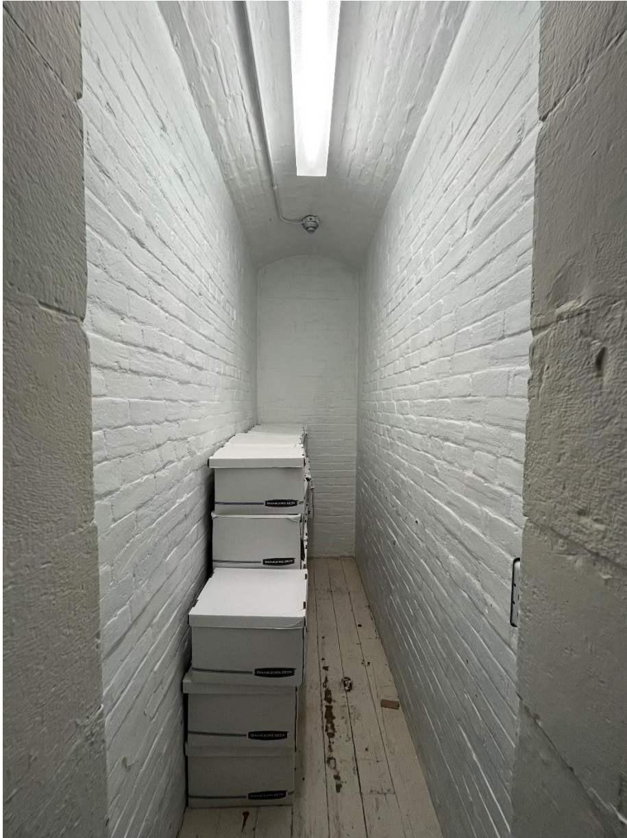
Figure 57: Example of a typical jail cell featuring barrel vaulted ceiling, brick walls, and wood floors. The size of the cell was determined by the occupant and nature of the crime committed, with similar sized cells grouped together (A.S.I., 2023).
