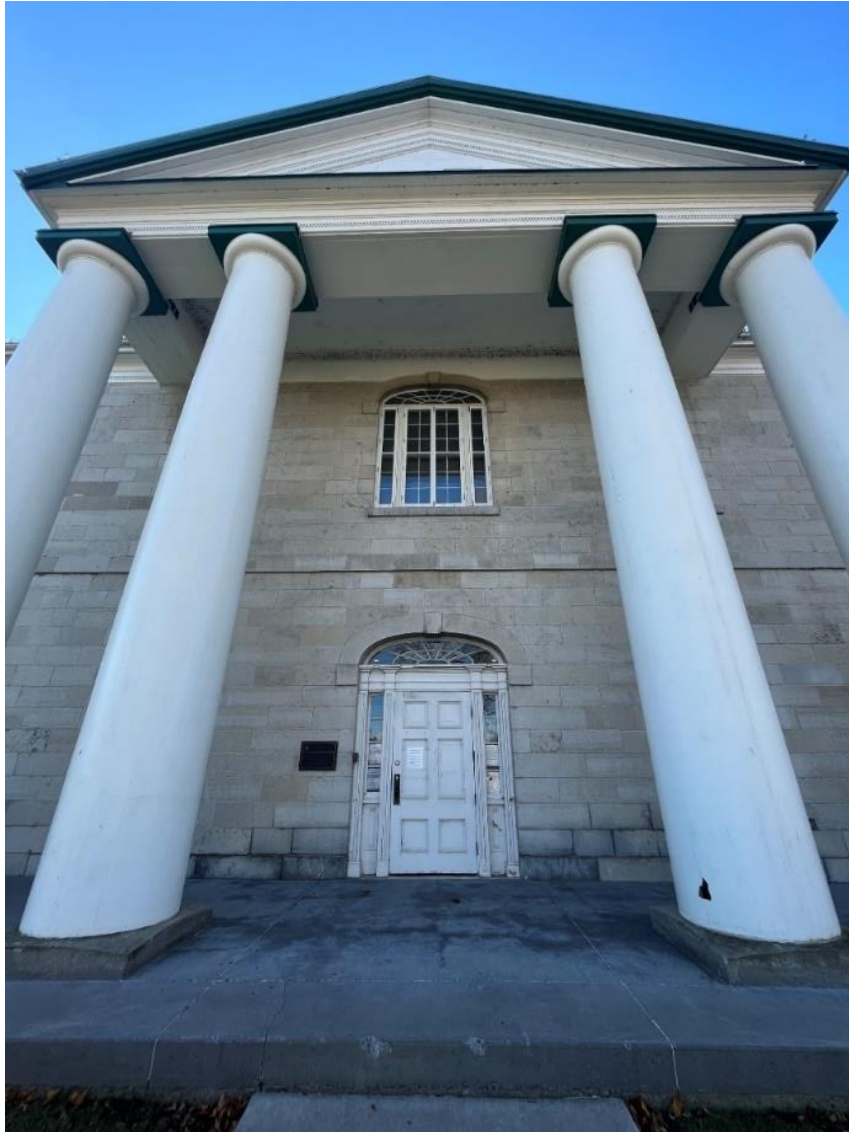
Figure 32: Detail of the portico added to the Georgian style courthouse by 1841. The giant order columns were replaced in 1993.
