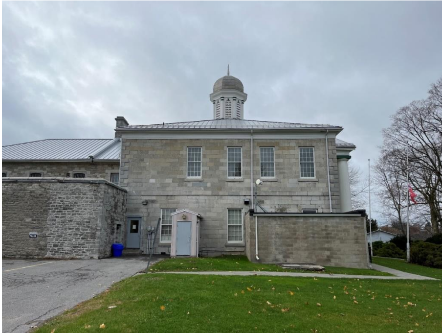
Figure 36: View of the east elevation showing the one storey concrete block addition and shed cover for the basement access (A.S.I. 2023).
