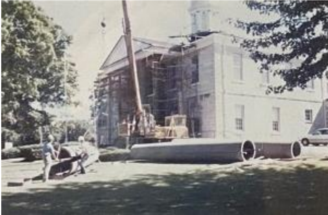
Figure 84: Replacement columns being prepared for installation within the portico of the courthouse in 1993 (Display board by M. O'lynn within the Picton Courthouse, documented by A.S.I., 2023).
