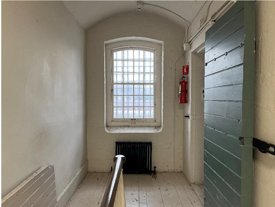
Figure 59: Detail of the second floor north corridor showing the original window, wood door, wood floors, and balustrade for the stairs leading to the first floor (A.S.I., 2023).
